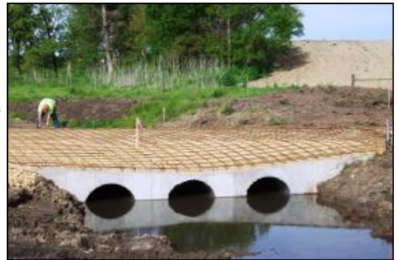
Low water crossing for Copper Creek
